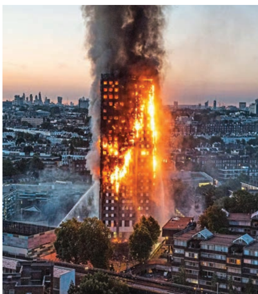
Pożar budynku Grenfell Tower, Londyn, 2017, źródło: https://www.standard.co.uk/news/london/revealed-the-dossier-of-deadly-failures-at-grenfell-tower-a3814871.html
